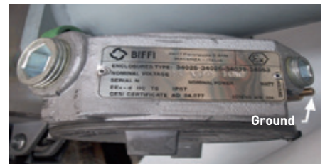
FIGURE 7 Junction box on control group (if foreseen)
