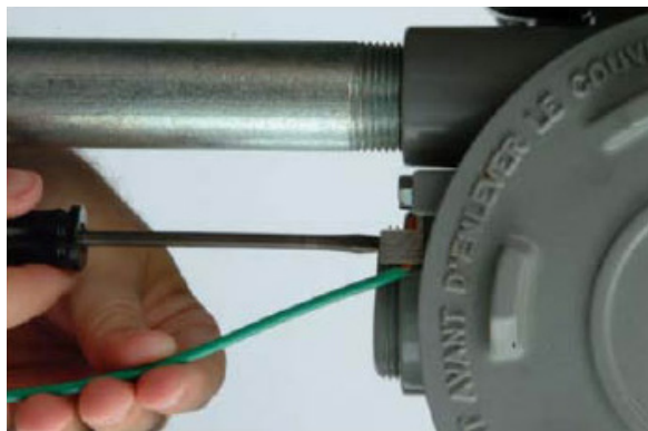
Figure 10. External Earth/Ground Connection
